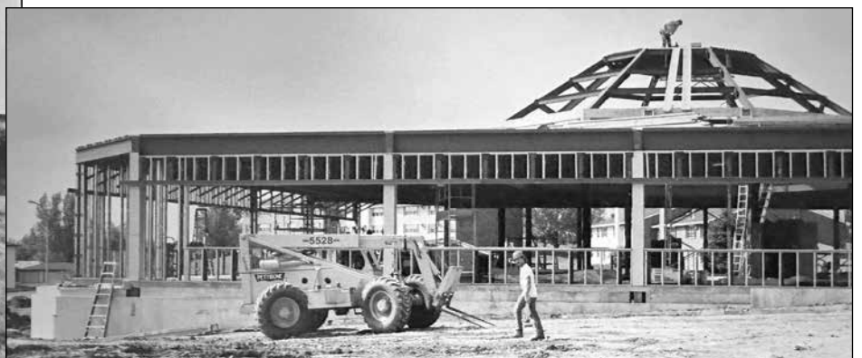
Ground breaking. NDACo headquarters construction – completed 2002.
